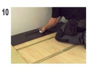
Connect the trap using the tightening tool provided, applying a bead of Jointing Compound around the neck of the tap.
