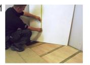
Carefully measure the Tapered Boards to fill the remainder of the wetfloor area, using Infill Panels where necessary.
