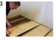
Cut and install 18mm plywood and fix onto the timber battens, to provide a support base for the wetfloor area finishing flush with the top of the joists.
