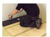
Screw the Drain Body intoplace using the pre-formed screw holes.
