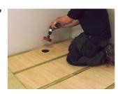
Using the pilot hole in the 18mm ply, cut a 100mm hole in the ply support for each trap.
