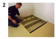
Check that all joists are level. Where necessary install noggins to support the edges of the wetfloor. Install timber battens 18mm from the top of the exposed joists.
