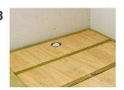
Remove the ply support and position the trap and connect to the wastepipe.
