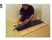
Where the grill is to be positioned against the wall, the Drain Body is trimmed to 220mm along the premarked 'cut line'
